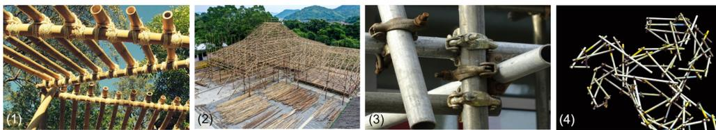
Figure 2: Examples of multi-tangent bar structures: (1) rope-lashed bamboo roof structures, (2) a temporary theater in Hong Kong made with bamboos, (3) construction scaffolding connected by swivel couplers, (4) a sculpture made out of scaffolding elements and couplers, by artist [Ben Long](#).
