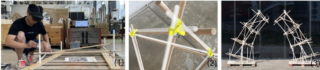
Figure 21: AR-assisted prefabrication of modules. (1-2) Workers are equipped with Hololens to see the spatial positions of the bars and couplers. The white bars are used for temporary reinforcement and support. (3) Two completed modules.
