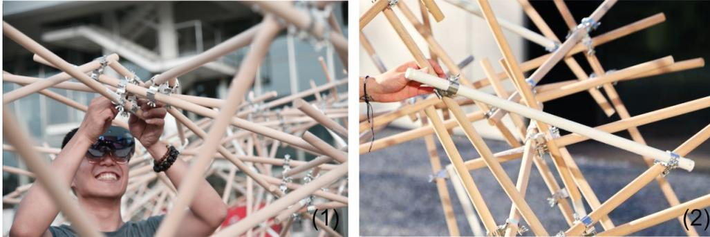
Figure 22: AR-assisted onsite assembly. (1) modules are transported on-site and assembled with AR guidance for accurate placement and connectivity. (2) after completion, the extra bars used for reinforcement (white bars) are removed.
