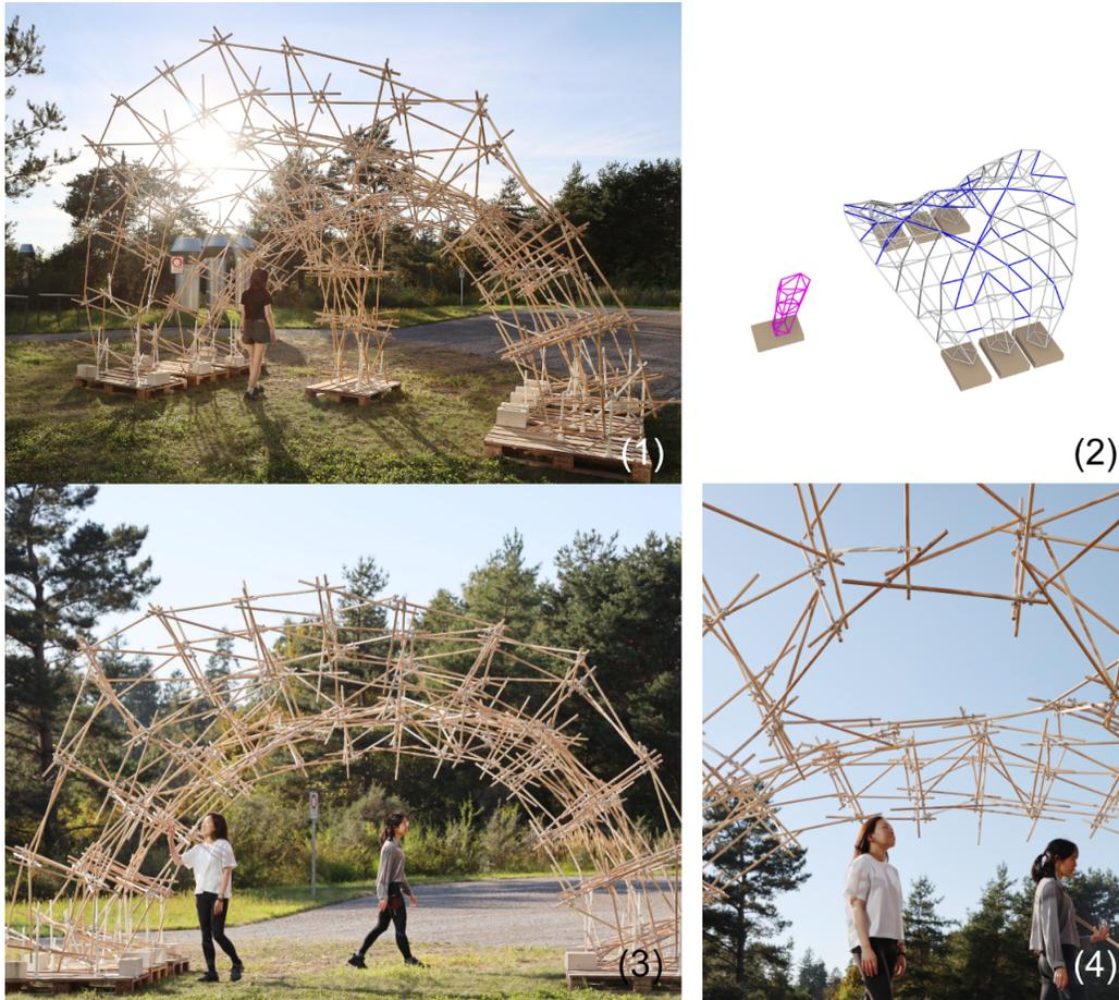
Figure 23: Archolumn is designed for two scenarios: with (1) and without the central column (3). Transformation is achieved by removing the central column (pink) and redistributing the bars to reinforce the arch (blue). While the structure before configuration shows a more enclosed, intimate space (1), the reconfigured structure provides a more open, spacious interior space that invites more daylight to come in (4).
